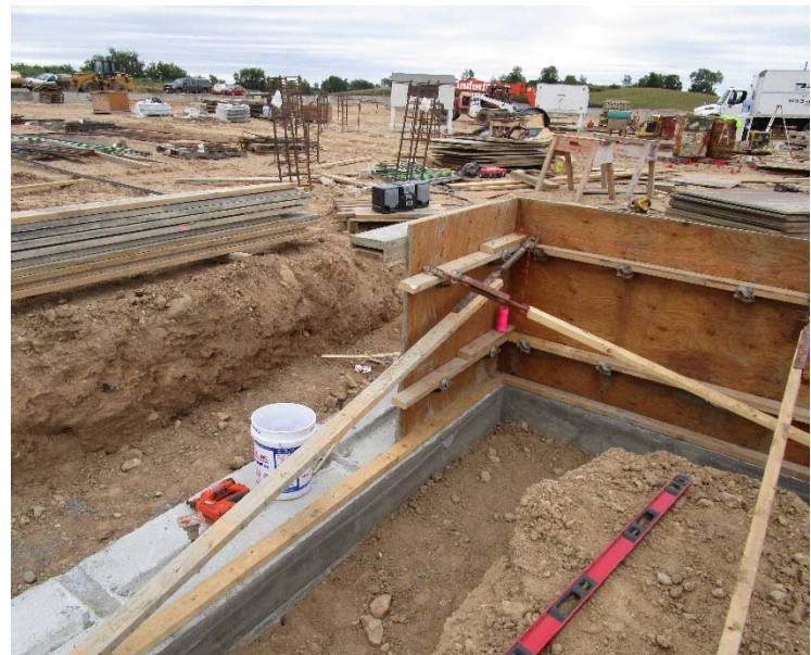
Area C's forms are being installed
