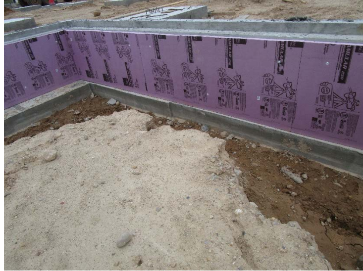
Exterior wall insulation installed on the foundation.
