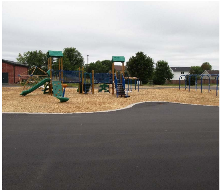
Asphalt surface course was placed, and the playgrounds are complete.
