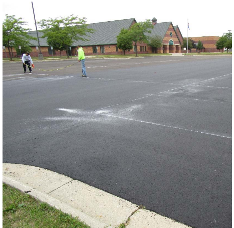
The front parking lot being prepped for striping.
