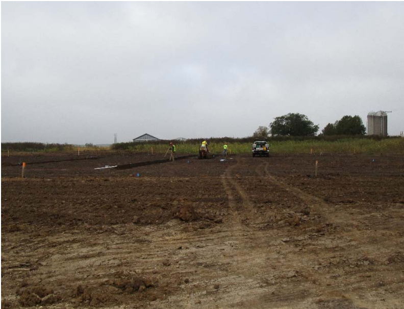
The Bruce Company installing irrigation in the new lacrosse field location.
