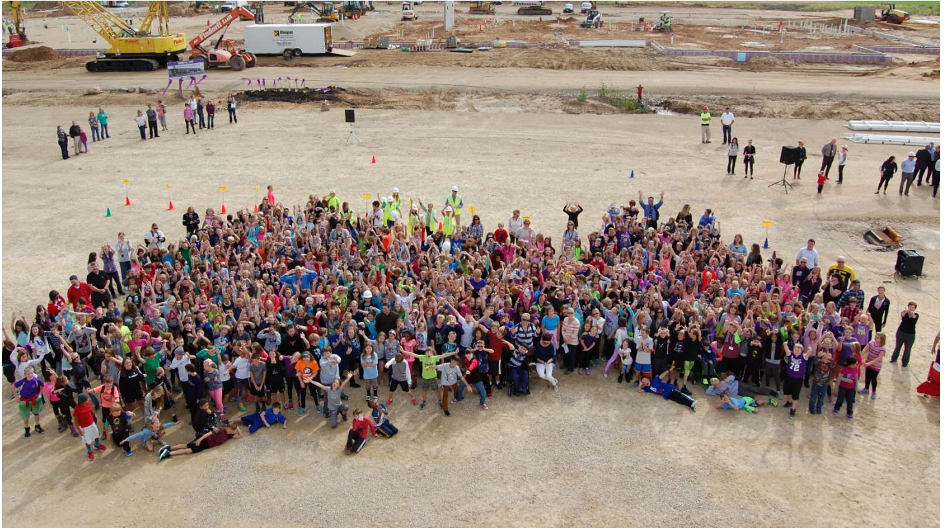
Our groundbreaking event was a huge success! Pictured here are all of the 4 th and 5 th grade students who will be the first to attend the New Intermediate School.
