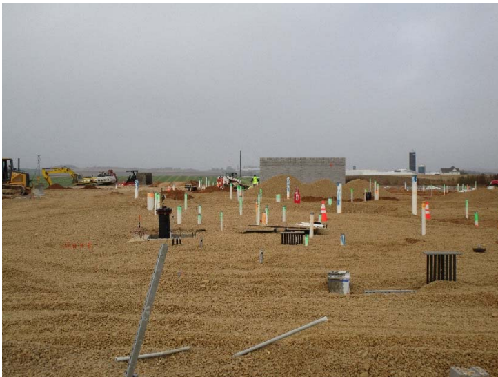
The building foundations and underground rough-ins were completed and filled to grade, and will be ready for steel and slab-on-grade next week.
