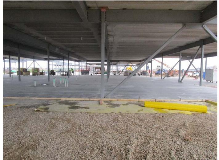
*The slab on grade that was poured in Area B under the plank. Future classrooms will be here!*
