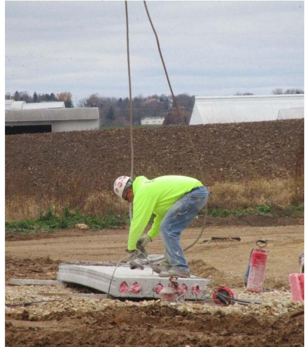
*A Findorff ironworker attaching the plank to the crane to be placed.*
