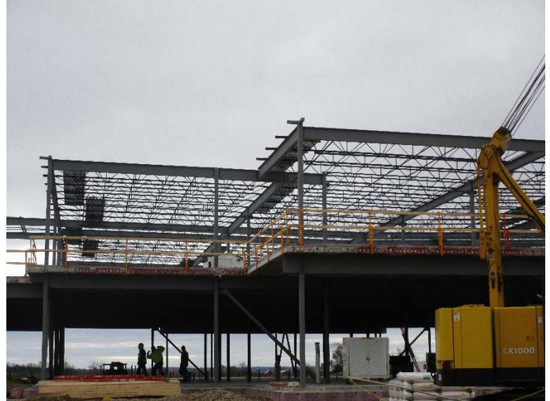
*Steel joists were installed this week, decking will start next week*
