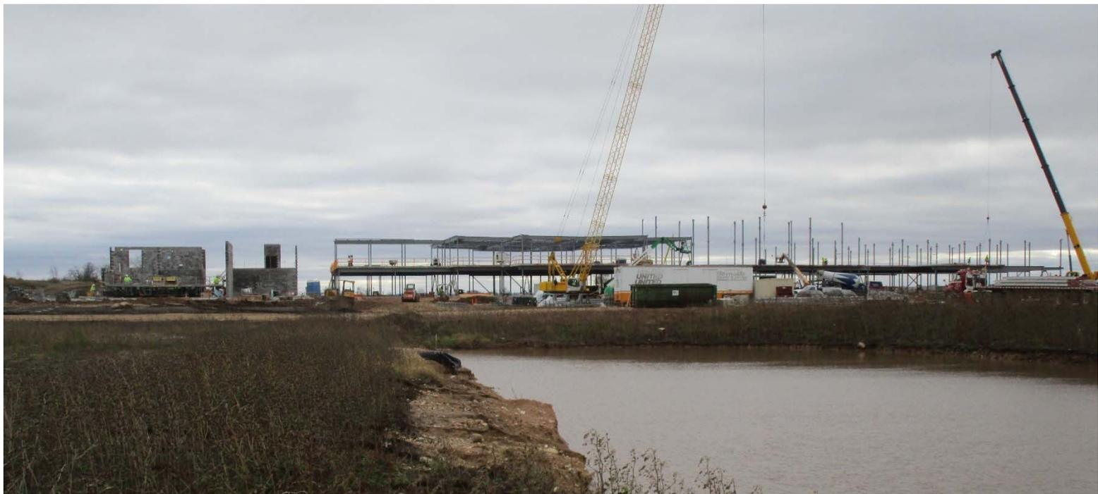
*In just two weeks, the building has more than doubled in size from the steel and precast plank decking! The music and main entry restrooms are taking shape on the left side of the photo.*
