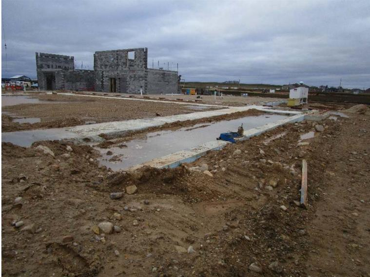
*Footings that will hold the precast gym panels in place. The panels will start being erected next week!*
