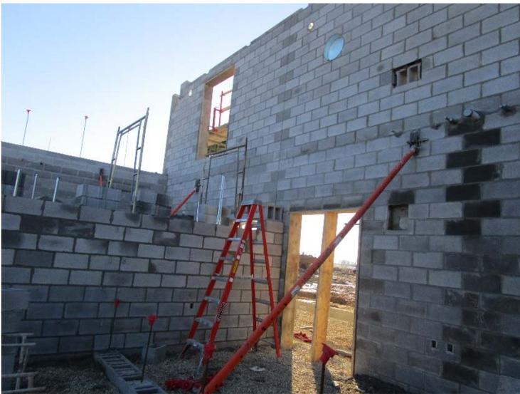
*Masonry has been moving quickly, with the bathroom and some of the music area walls set up to the second floor.*
