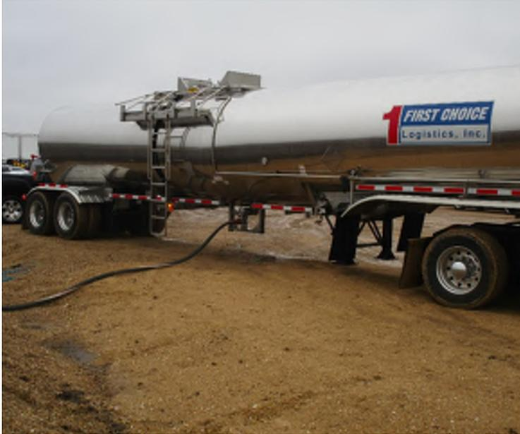
Multiple semi trucks full of glycol getting pumped into the geothermal system through the vault. This will keep the lines from freezing when circulating between the geothermal field and the building.
