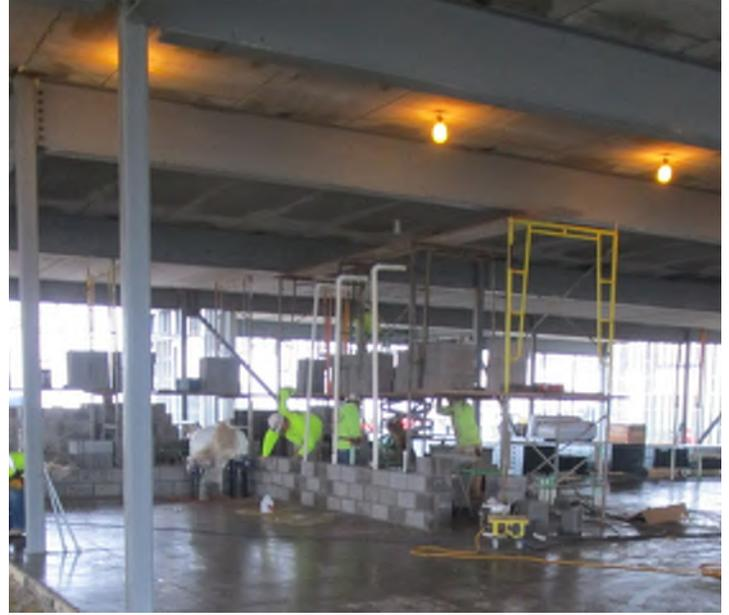
Interior masonry is moving along, with a lot of Area 2B completed, the masons were able to move to the first floor to start work.
