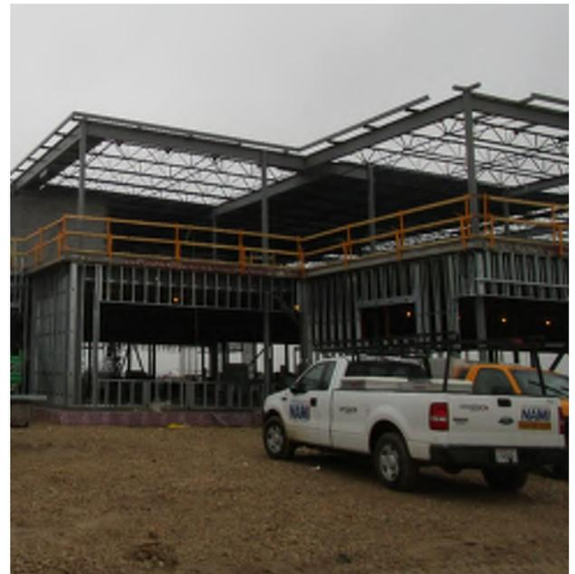
*Steel decking started installation this week in preparation for roofing in the coming weeks.*
