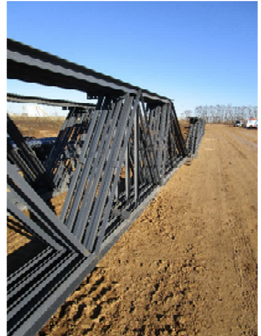
The large gym joists arrived onsite this week.
