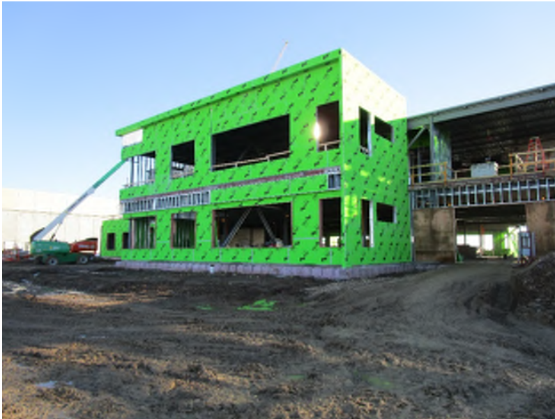
Area B exterior studs with a layer of dens glass installed.
