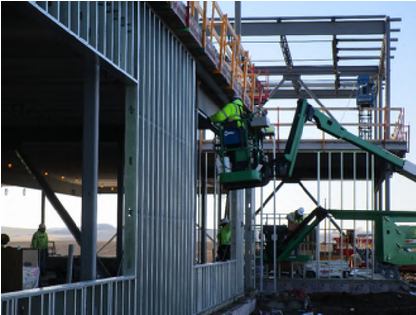
A Findorff carpenter installing studs in area B.
