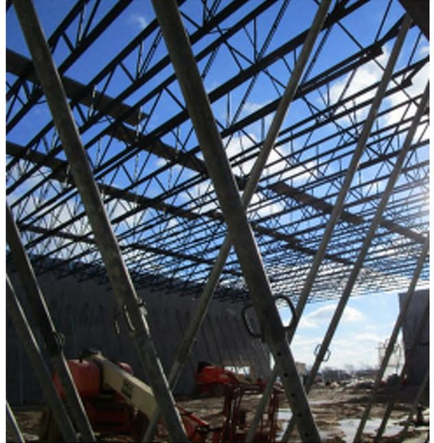
*The large gym joists were installed last week in just 3 days!*
