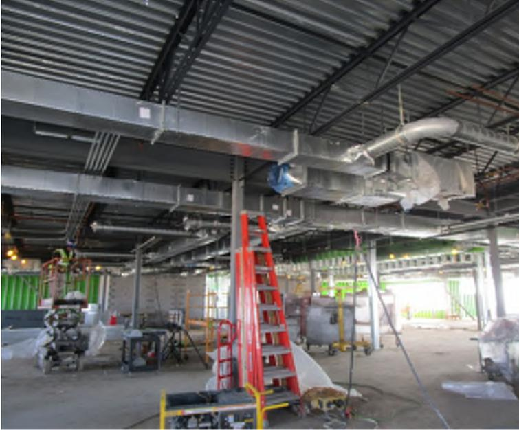
*Most of the ductwork in Area B has been completed as shown, and they have moved to the first floor.*
