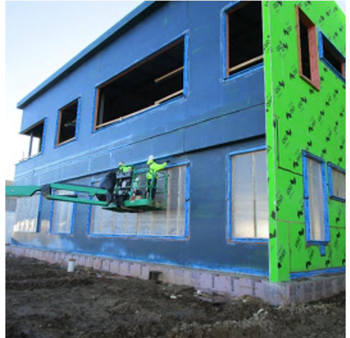
*Dens glass with a layer of weather barrier applied. Temporary window enclosures installed on the windows.*
