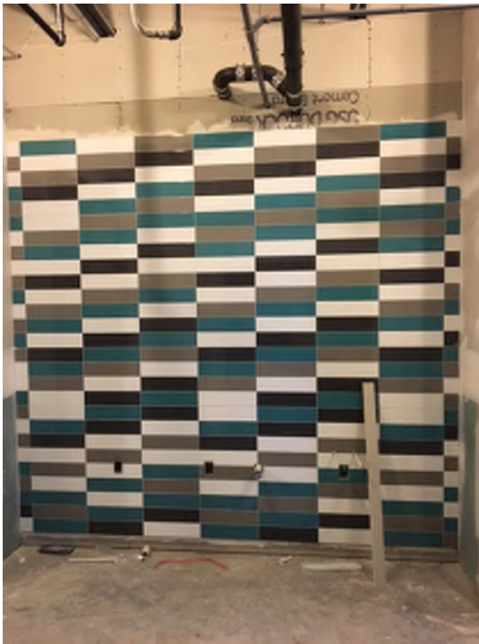
Wall tile outside a 2B restroom shows an aesthetic pattern and the color designates the Village you are in
