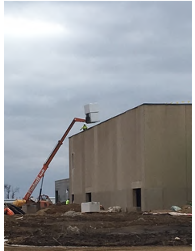
A telescoping fork lift hoists roofing materials onto the gym.
