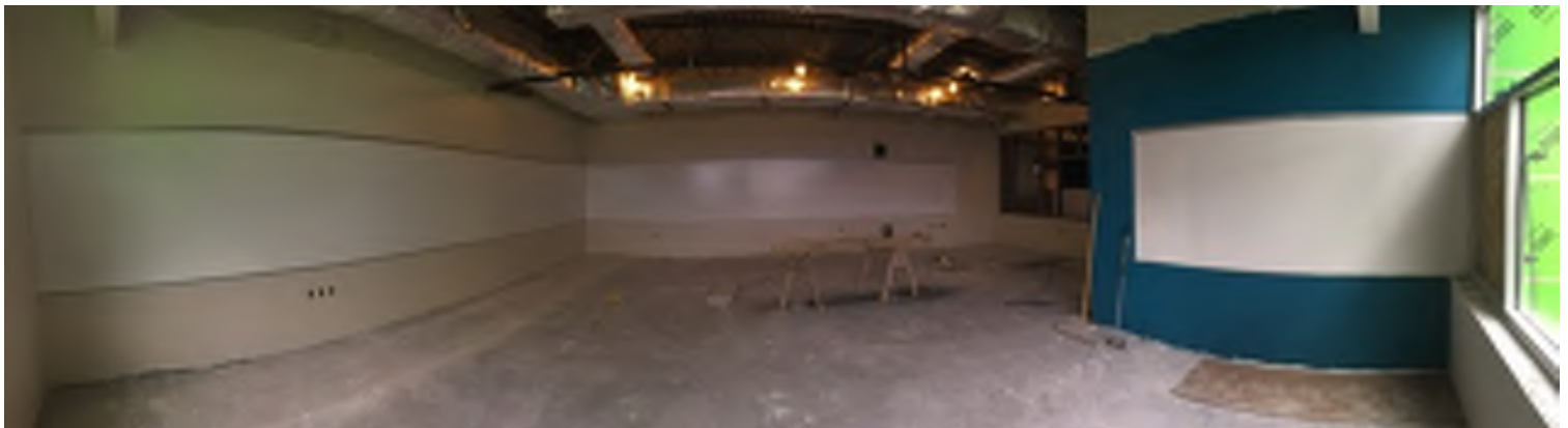
Panoramic view of a typical Learning Environment Room. Markerboard walls surround the room and are painted out for review. This classroom is in south side of Area 2B.
