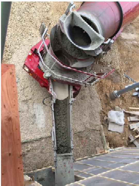
Birds eye view of a concrete pour in Area C.
