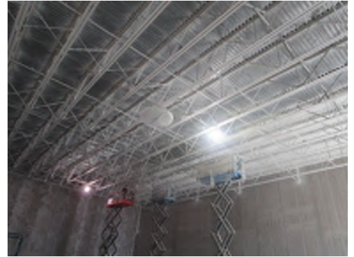
Gym ceiling being painted.
