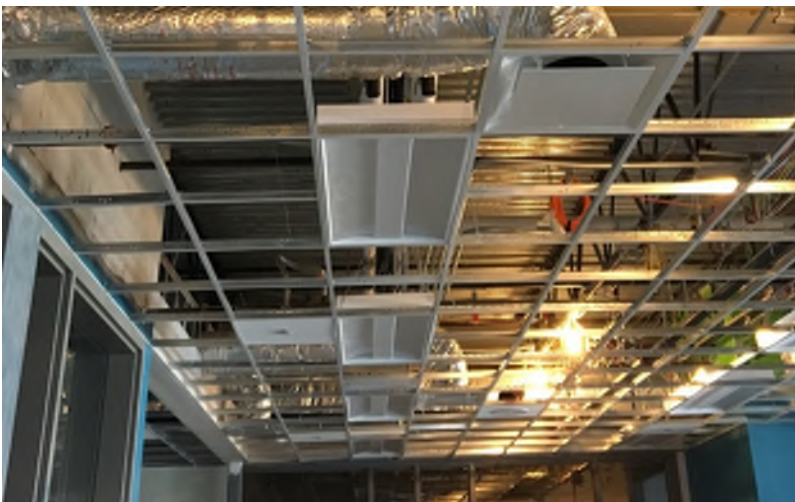
Light fixture installation continues on 2 nd floor
