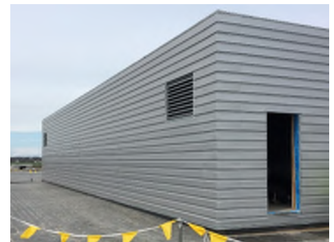
Silver metal panels placed at the area A mezzanine
