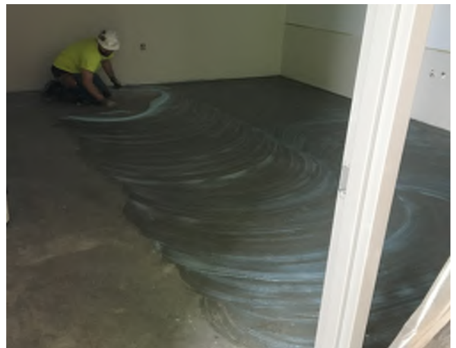
Prep for carpeting includes spreading adhesive as pictured above
