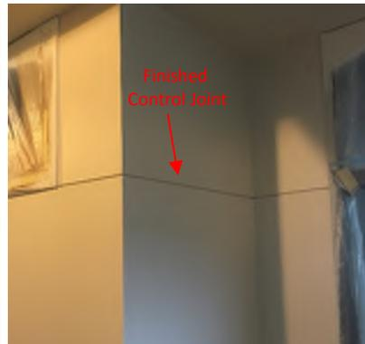
*The two pictures above show a corridor wall before and after the finishes were completed. The white strip of plastic running horizontally is called a Drywall Expansion Joint or Control Joint. This prevents cracking in the gypsum board that occurs from drywall expansion.*
