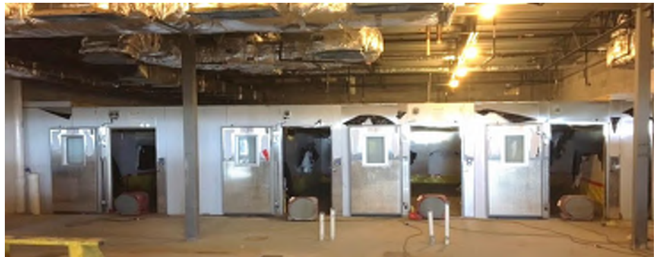
A full four-door fridge/freezer was recently installed in the kitchen
