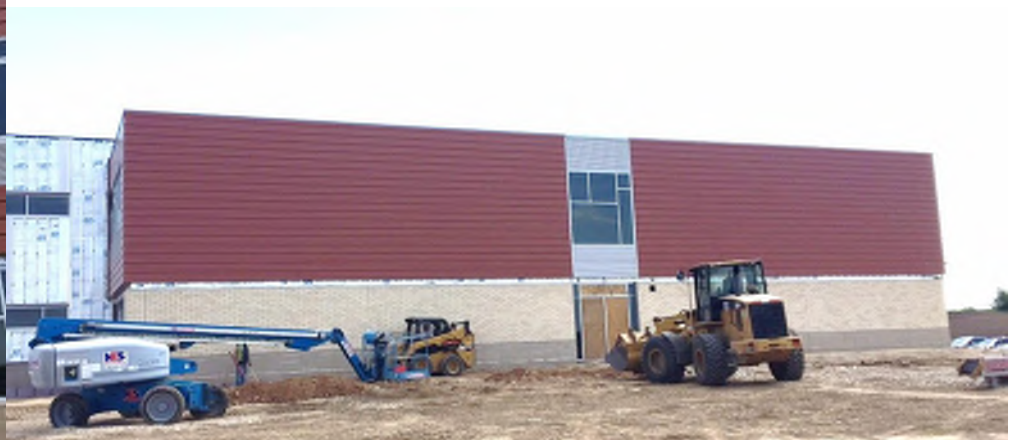
Take a look at the new redwood metal panels. They will cover the west elevation (above) along with all the recessed areas around the exterior of the building (left).
