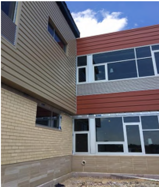
Take a look at the new redwood metal panels. They will cover the west elevation (above) along with all the recessed areas around the exterior of the building (left).
