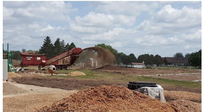
It is pretty interesting to see how the amended soil is spread. It looks almost like they are using a giant snow blower!
