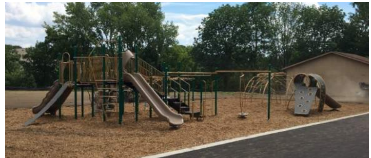
Playground equipment install finished up this week.
