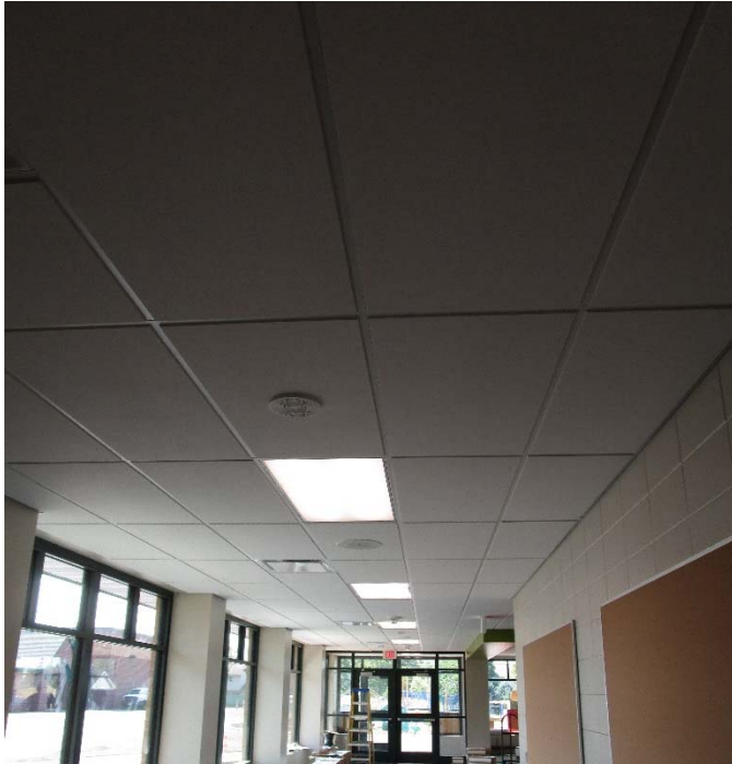
The completed ceiling at the new kindergarten addition.
