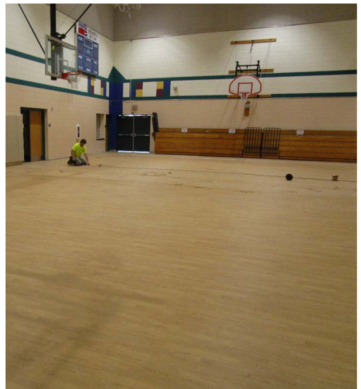
Finishing touches to the new gym floor.
