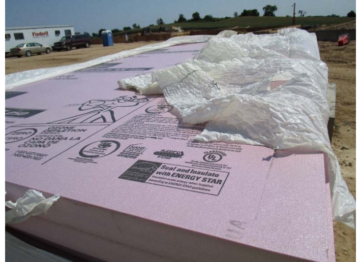
Exterior wall insulation prior to installation.
