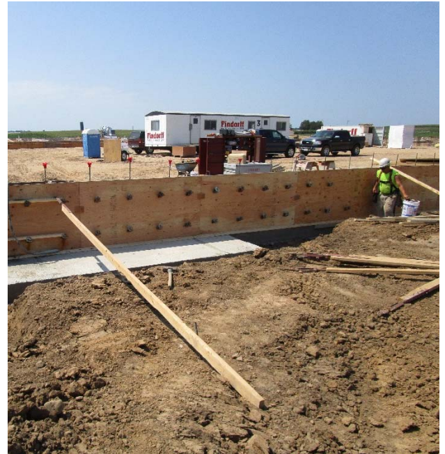
Carpenters working on the forms for the Area C foundations.
