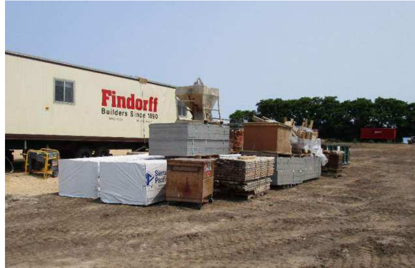
Materials needed for foundation work are beginning to arrive
