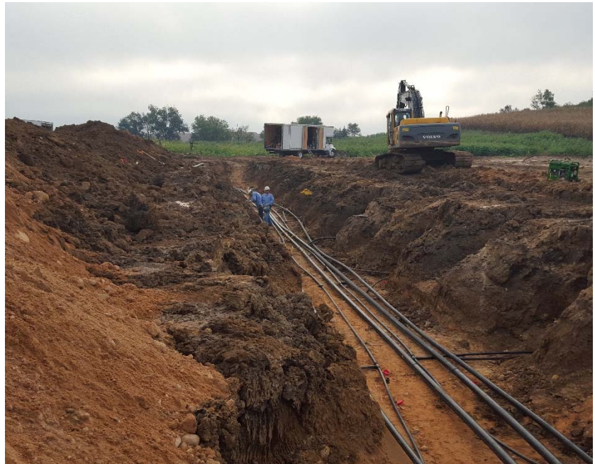
Completing the loops for the geothermal system.
