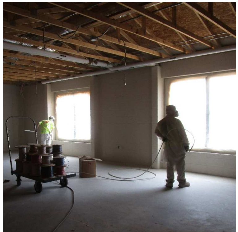
Painters working hard to make the addition look like a classroom.
