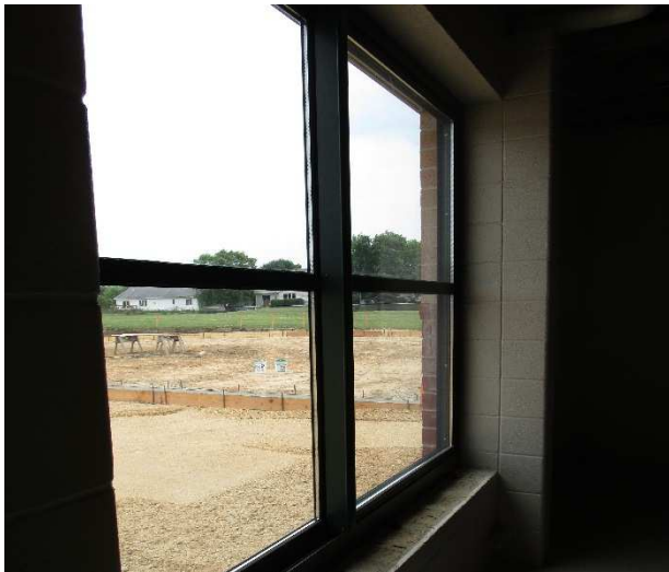
New windows in the addition.
