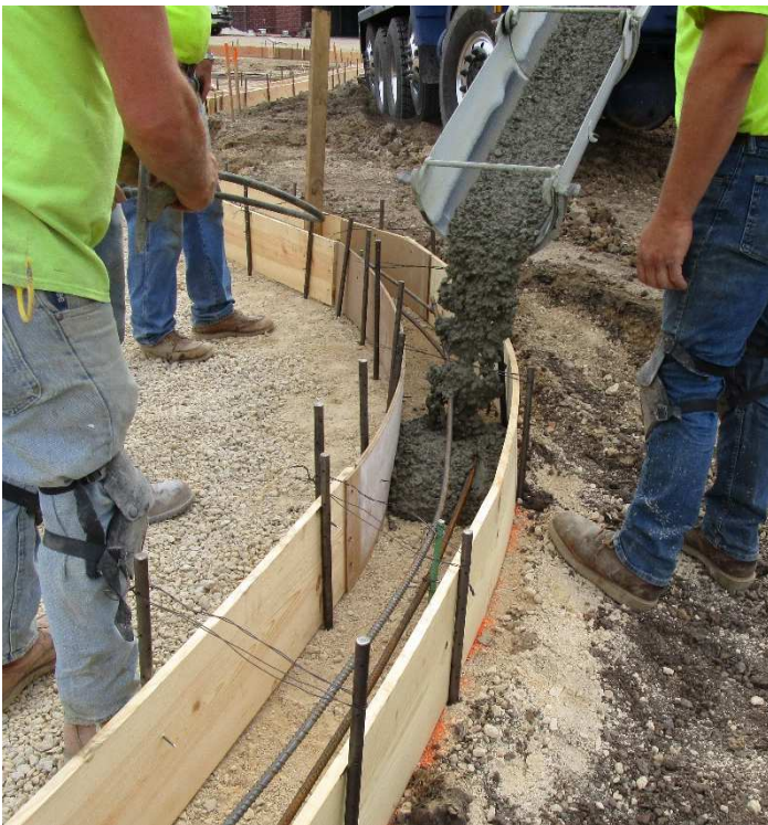
Concrete being poured around the perimeter of the new playground area.
