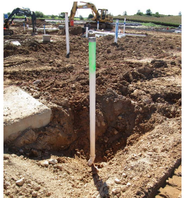
Green tops will be used for sanitary sewer transportation.
