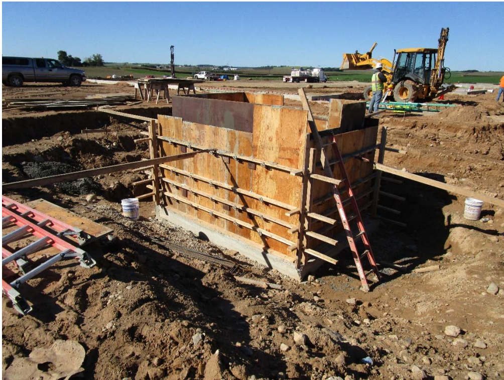
Elevator pit form for future elevator.
