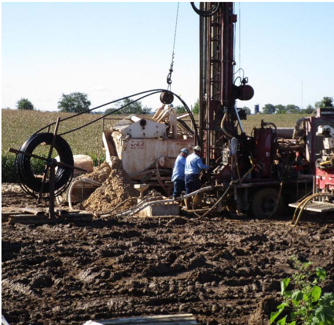
Geothermal drilling is still making good progress.
