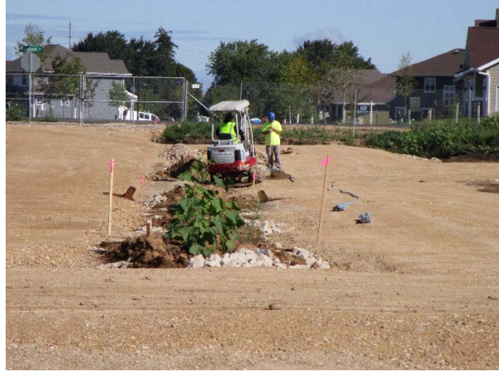
Westphal laying out locations for site conduit
