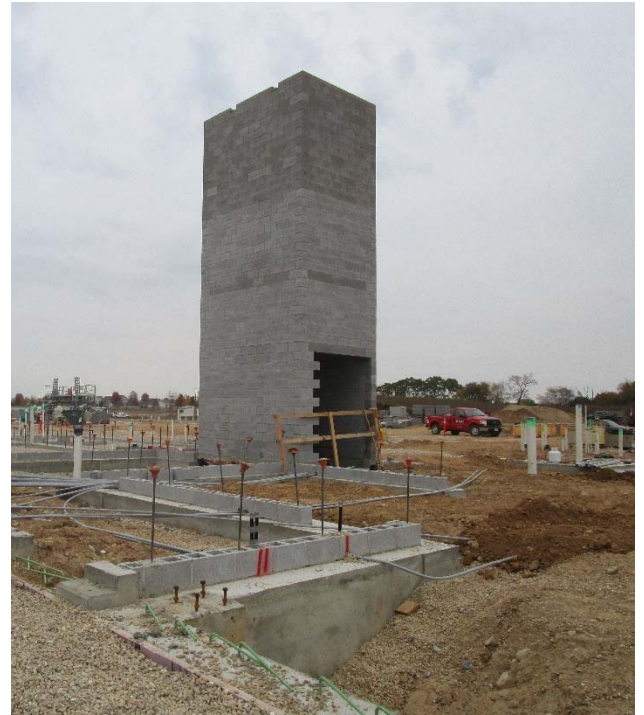
The masons completed the elevator shaft this week.
