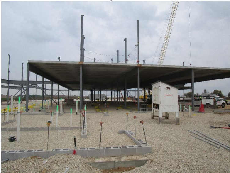
Structural steel and precast plank up to the second floor.
