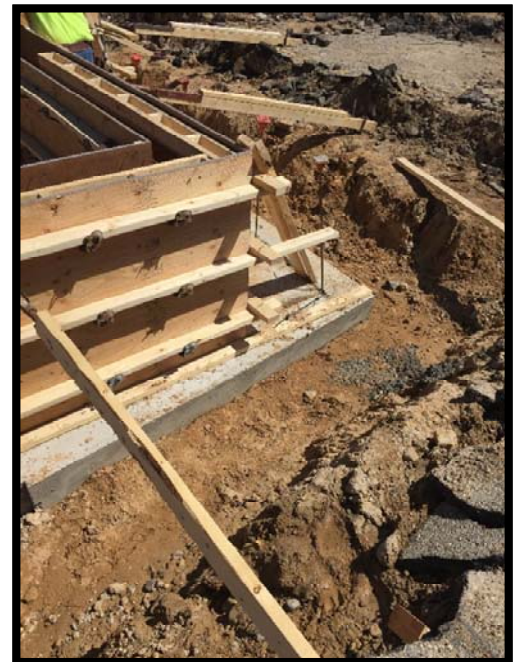
Wall forms constructed by Findorff crew.
