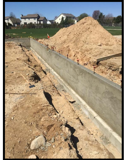
Northern foundation walls that were recently poured.
