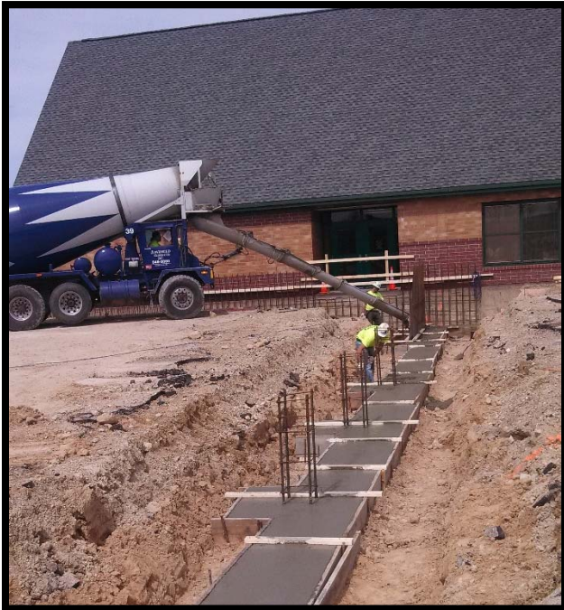
Findorff crew members pour footings.
