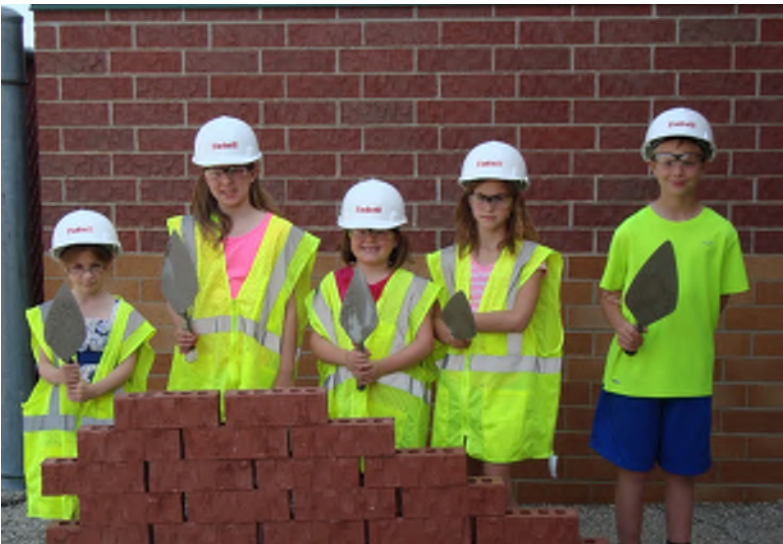
A student from each grade level was selected to participate in laying brick for the new addition! Thanks for your help!
