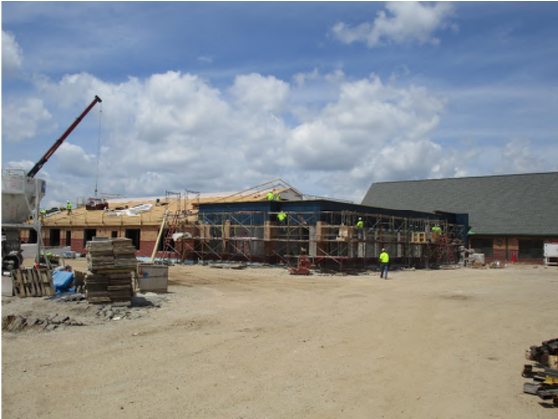
The exterior progress of the new addition.
