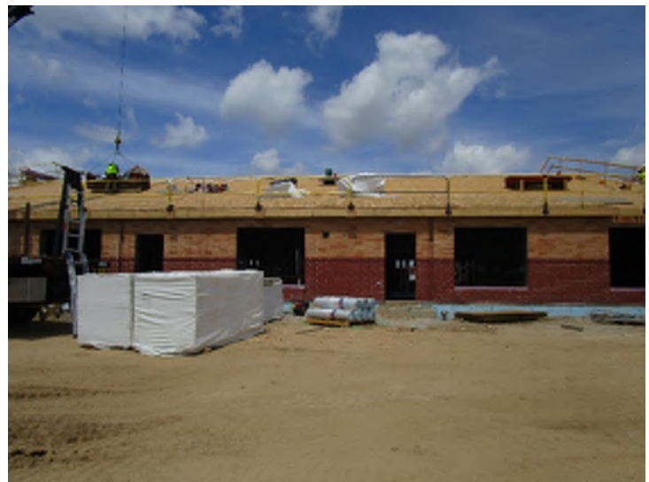
The roof is being prepped for insulation and shingles.
