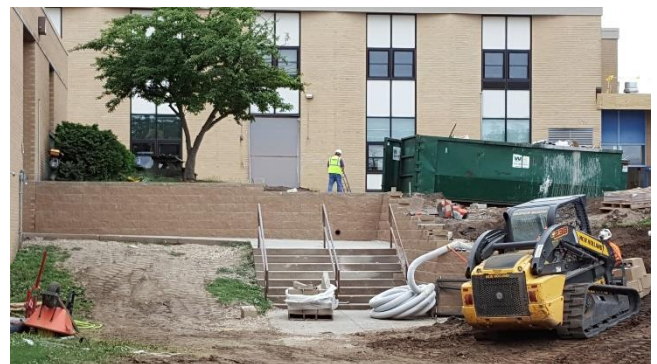
The new retaining wall is off to a great start!
