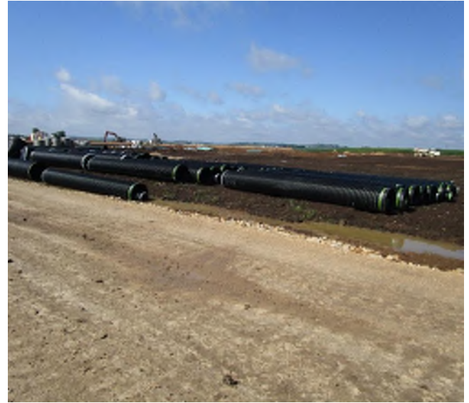
Site utility materials waiting for installation.
