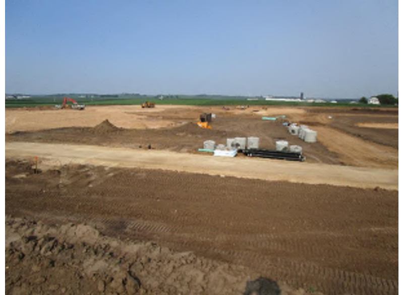
Progress of new building location, along with delivered materials.
