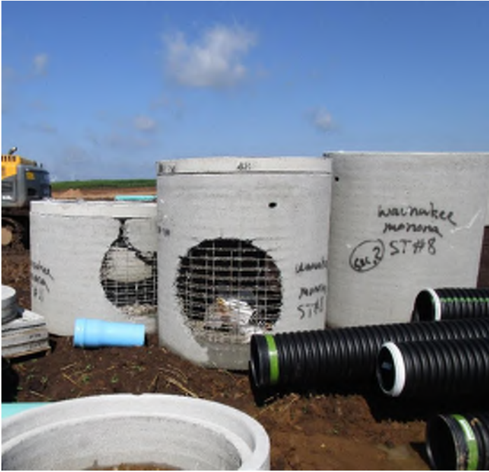
Storm structures were delivered to the site for install
