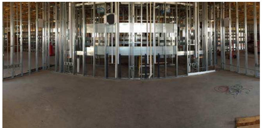
One of the new breakout areas, ready for drywall!
