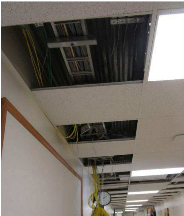
Some of the electrical work taking place in the existing school
