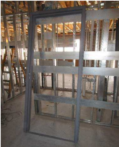
Hollow metal frames to be installed just before the drywall.
