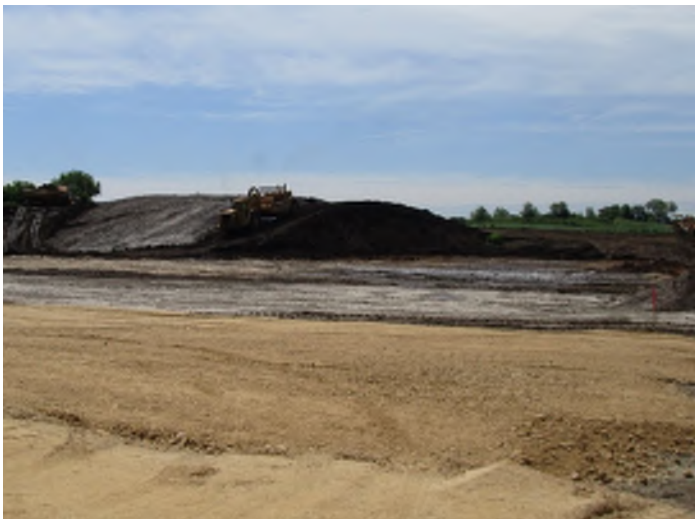
Earthmovers are removing the topsoil and stockpiling.
