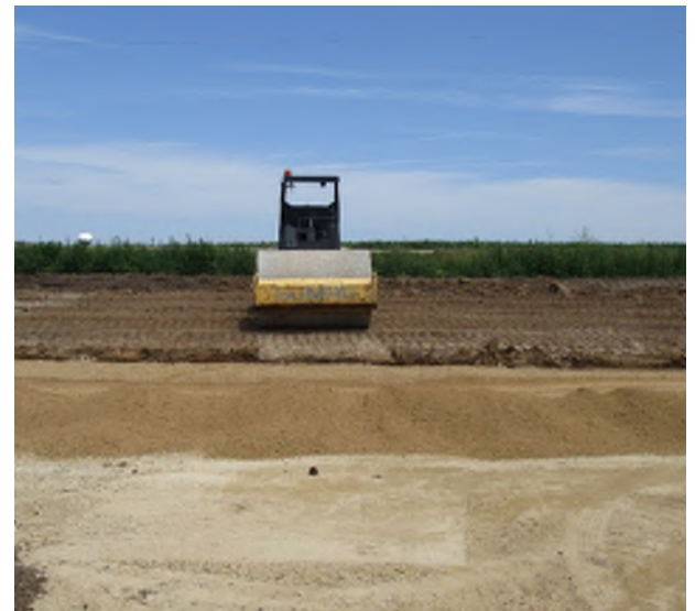
Compactor onsite to get the roadway established.
