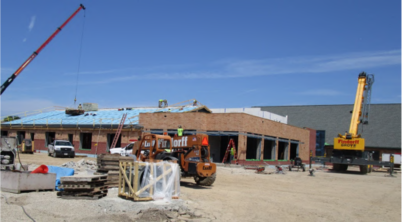
The exterior brick is done and it looks great!
