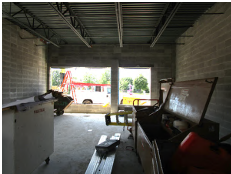
The flat roof is finished in the new addition breakout area. Also pictured is the windows prepped to be watertight.
