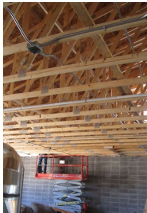
Electrical subcontractor installing conduit.
